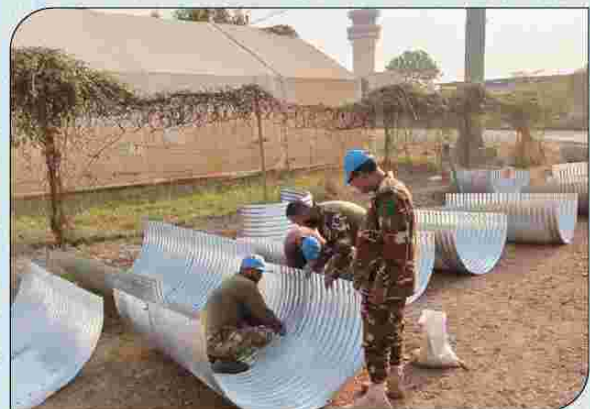
Construction of open steel culverts in Tumping by BANCEC-23, UNMISS, Sudan
