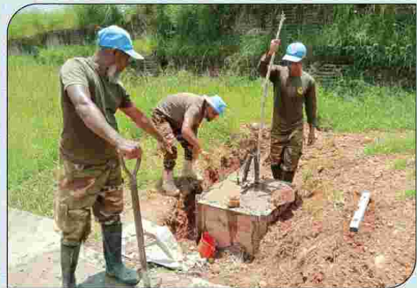
Construction of foundations and trenching for security lights along durupi Camp Perimeter by BANENGR (RPF) COY/7, UNMISS, South Sudan
