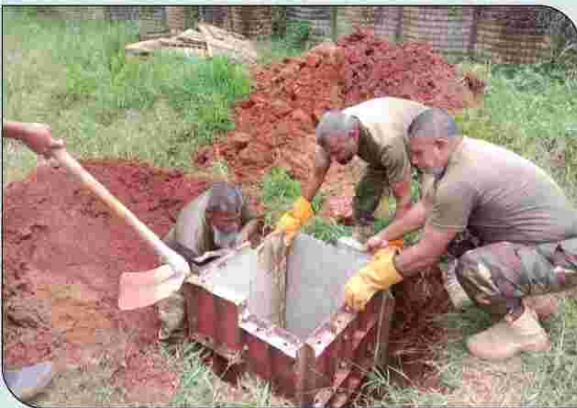
Construction of foundations and trenching for security lights along durupi Camp Perimeter by BANENGR (RPF) COY/7, UNMISS, South Sudan
