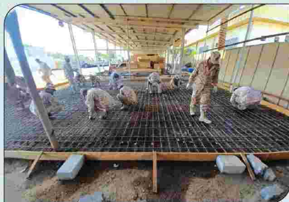
Floor Rebar binding of parking shed at Military Police Unit, Gewan
